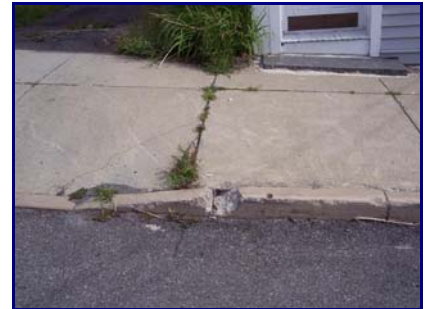
Sidewalk and curbing repair needed.
